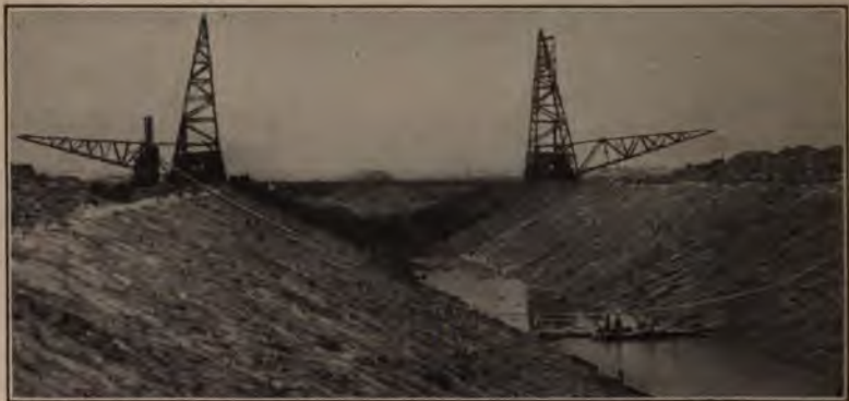
Double Tower Excavator. Figure 70.
